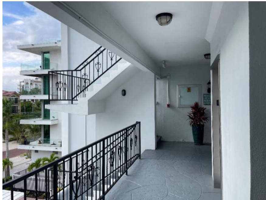
Figure 13: Typical walkway area observed.
