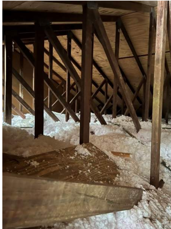
Figure 19: Attic and trusses
