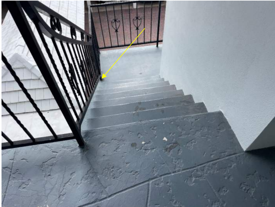
Figure 14: Typical stairwell overview.
