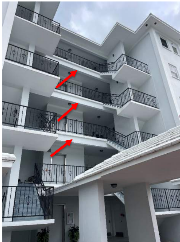
Figure 4: Typical Concrete Beams Observed.
