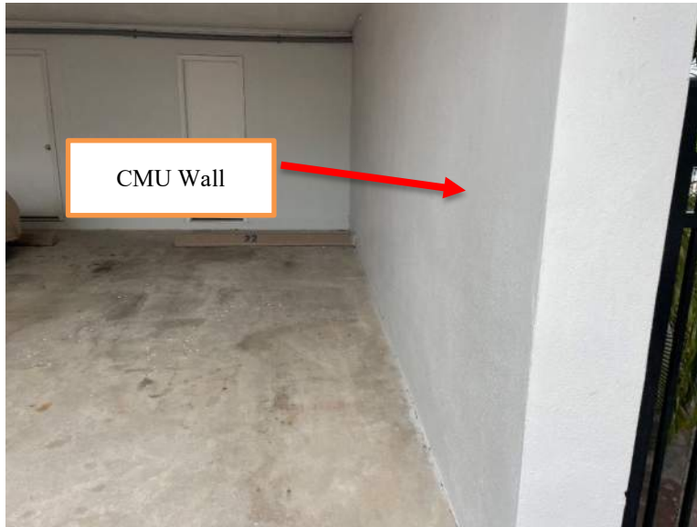
Figure 7: Example of CMU wall connected to an exterior column
