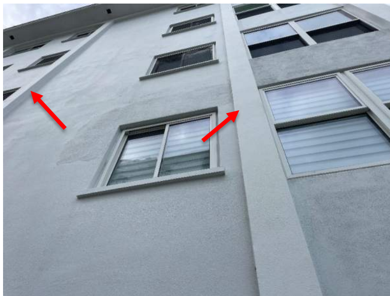
Figure 5: Typical columns observed.
