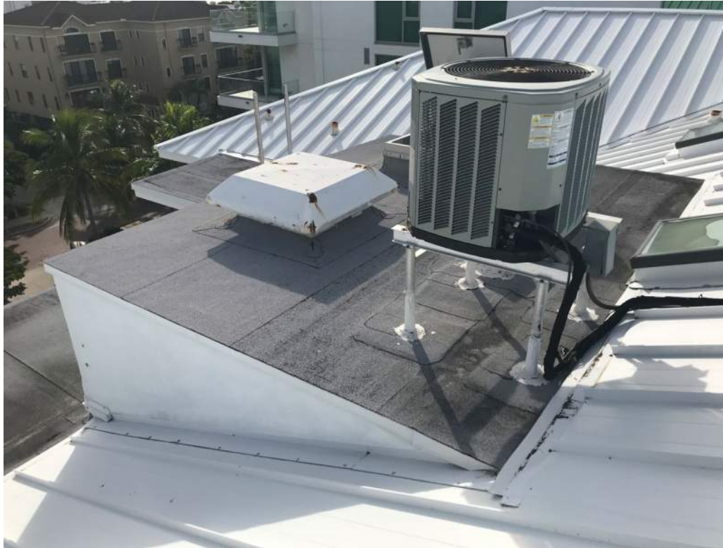
Figure 18: Roof existing condition
